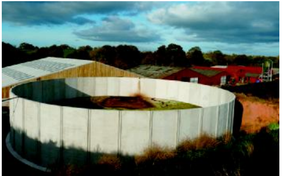
To cater for the proposed herd expansion a new 2.5m litre slurry store has been build.
